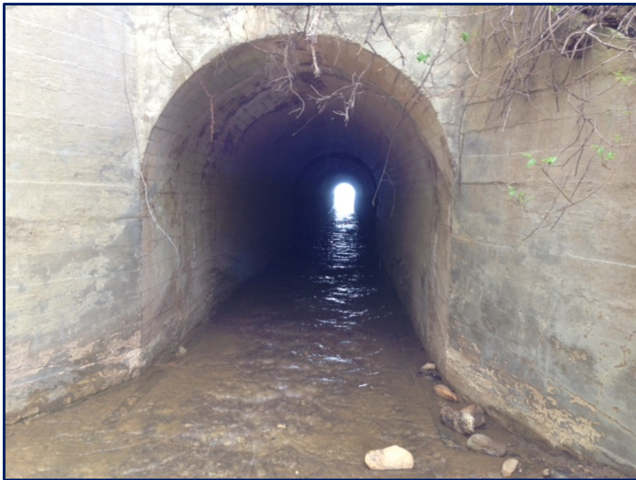
Entrance to tunnel
